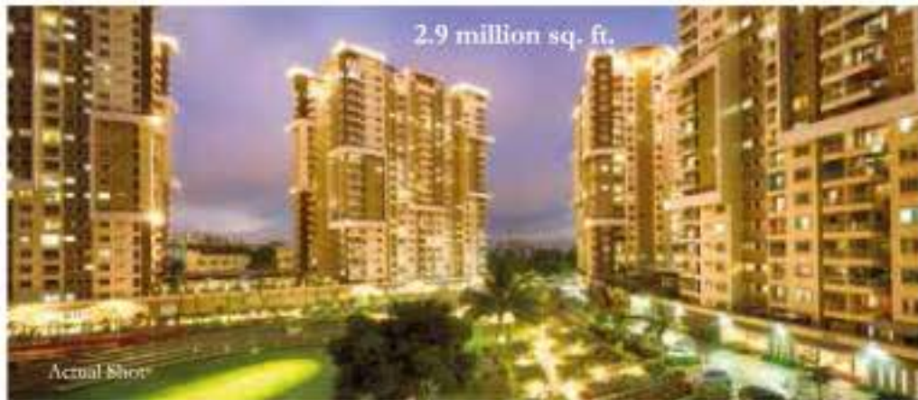
GREENAGE Hosur Main Road
