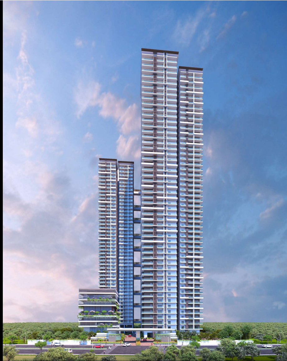
Proposed Residential Apartment "ALTUS" Developed by M/s. HallMark Infra Heights LLP at Kondapur, Hyd.
