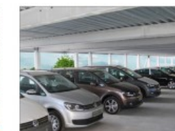
Covered Car Parking
