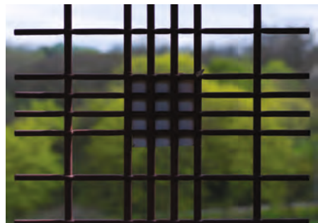
Security Grills on windows
