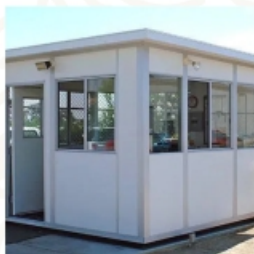
Watchman Room and Common Toilet
