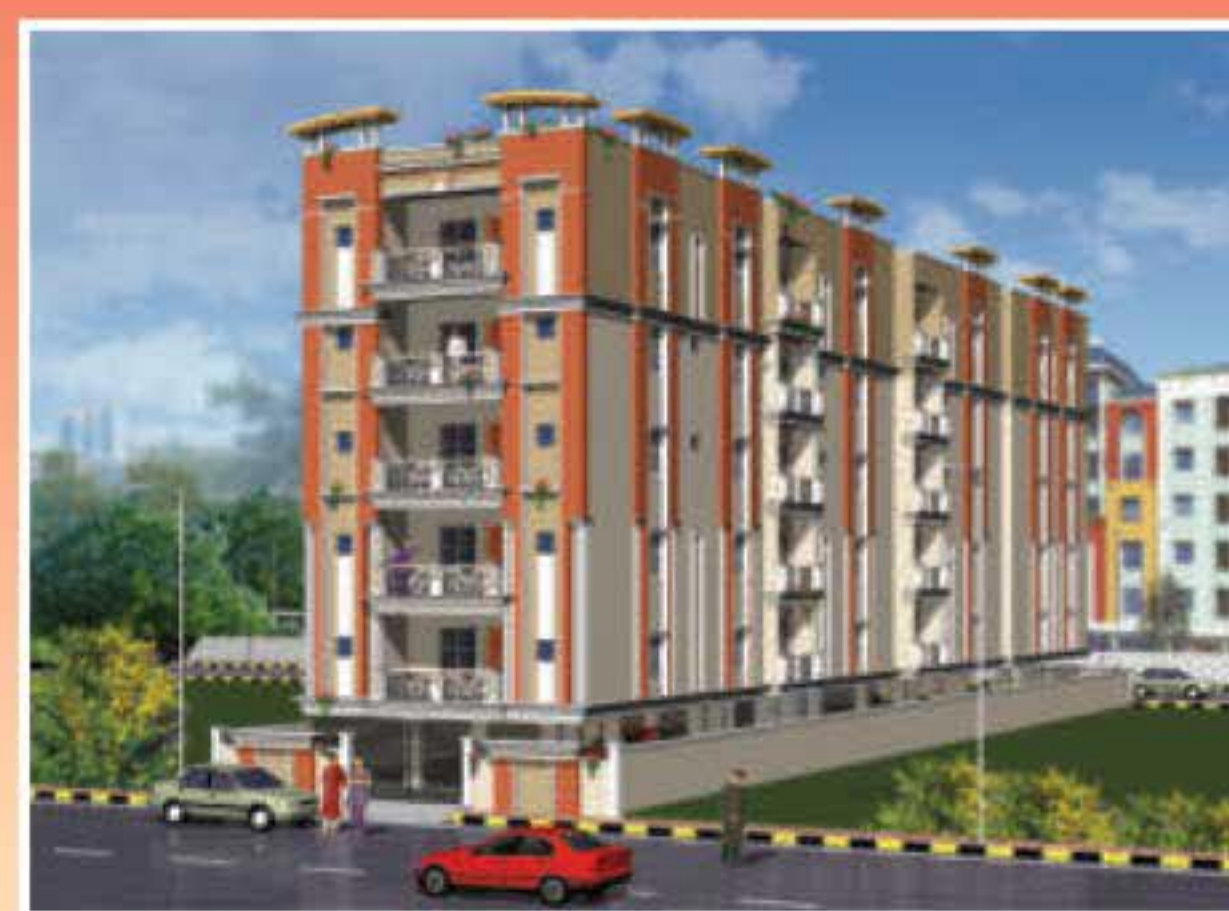
Surya Pearl at Gandhi Nagar
