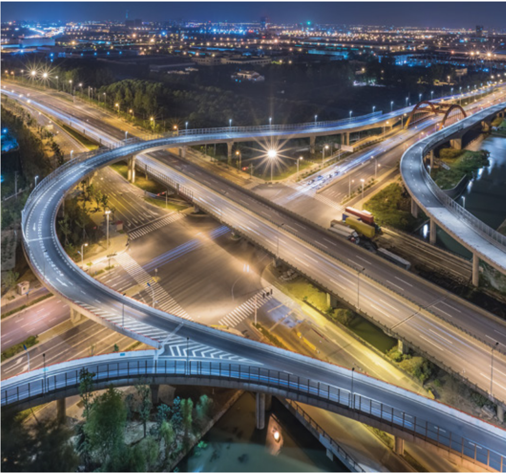
Goregaon–Mulund Link Road (GMLR)
