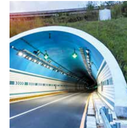
BORIVALI - THANE TUNNEL
