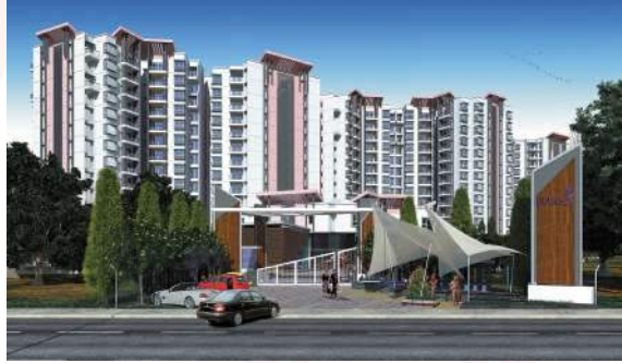
Running Project: Durga Petals Marathahalli, Bengaluru - 560037
