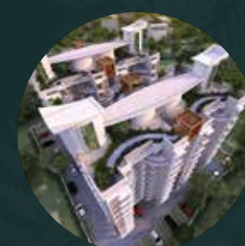
Protech Green Panjabari, Guwahati, Aug'20 (Ongoing)
