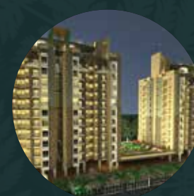
Protech Paradise Kahilipara, Guwahati, Aug'20 (Ongoing)
