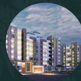
Protech Galaxy Bhetapara, Guwahati, Jan'18 - Completed on 30th Oct'21
