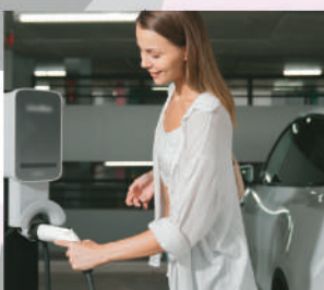
EV CHARGE POINT AT CAR PARKING
