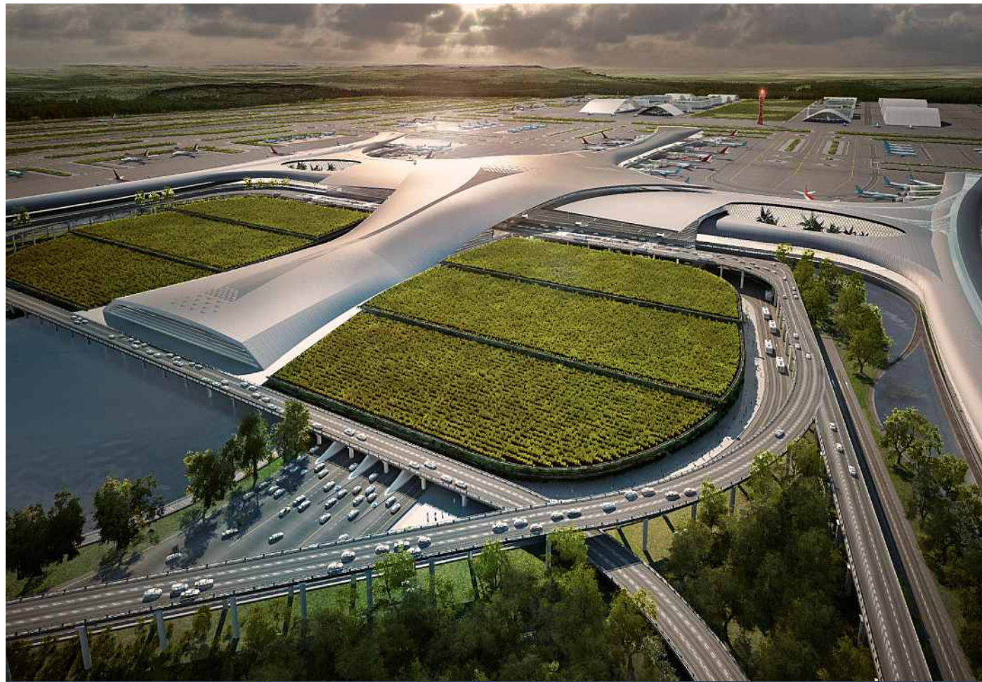
Qingdao New Airport, China
