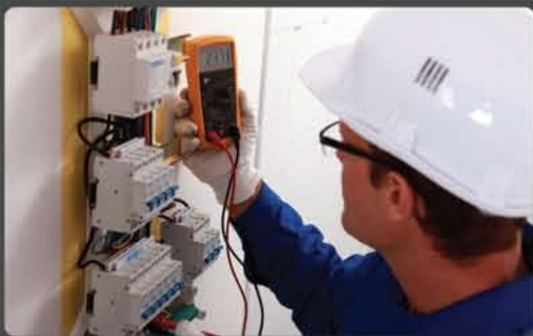
Electrical Adequate Electric points, Intercom facilities. Regulated entry with Intercom Connection from Entrance Gate to each Apartment. Fire resistant electric wires with elegant modular switches.
