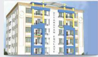
Uttarayan Enclave, Beltola Survey Road, Guwahati
