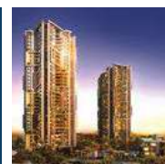
Apartments Villas Integrated Enclaves Senior Living
