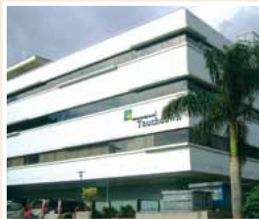
TOUCHDOWN COMMERCIAL BUILDING NEAR HAL INDUSTRIAL AREA, BANGALORE
