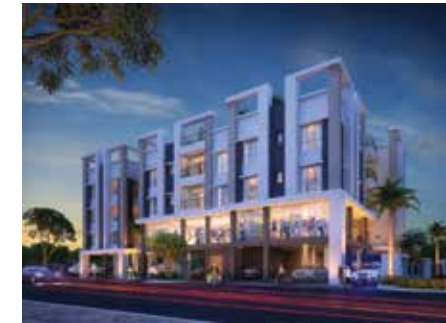
Ekam Solace near Park Street
