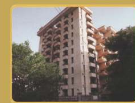
Khattar Co-operative Apartments Consisting 100 units
