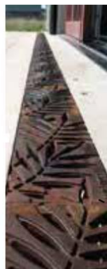
Ornate cast covers on all visible drains.
