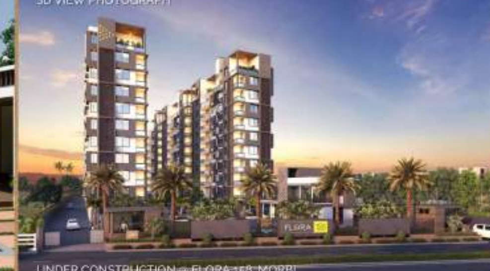
UNDER CONSTRUCTION @ FLORA 158, MORBI
