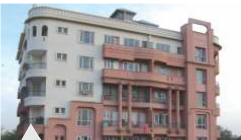
SIDDHA TOWER Residential Apartments Banipark, Jaipur
