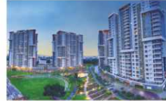
GREENAGE Hosur Main Road, Bengaluru
