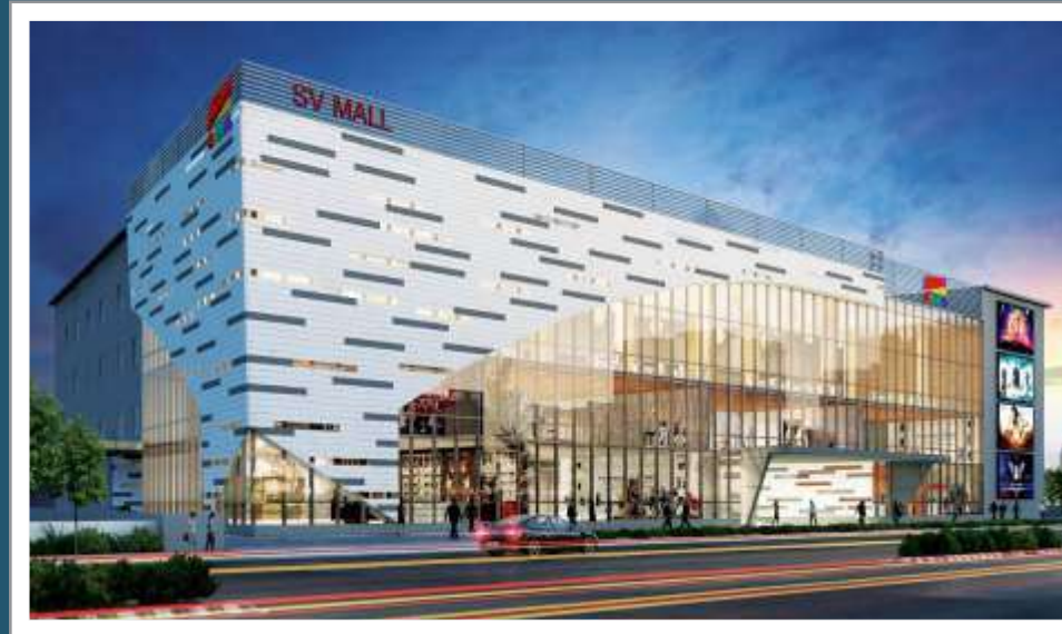
SV Mall @ Adibatla
