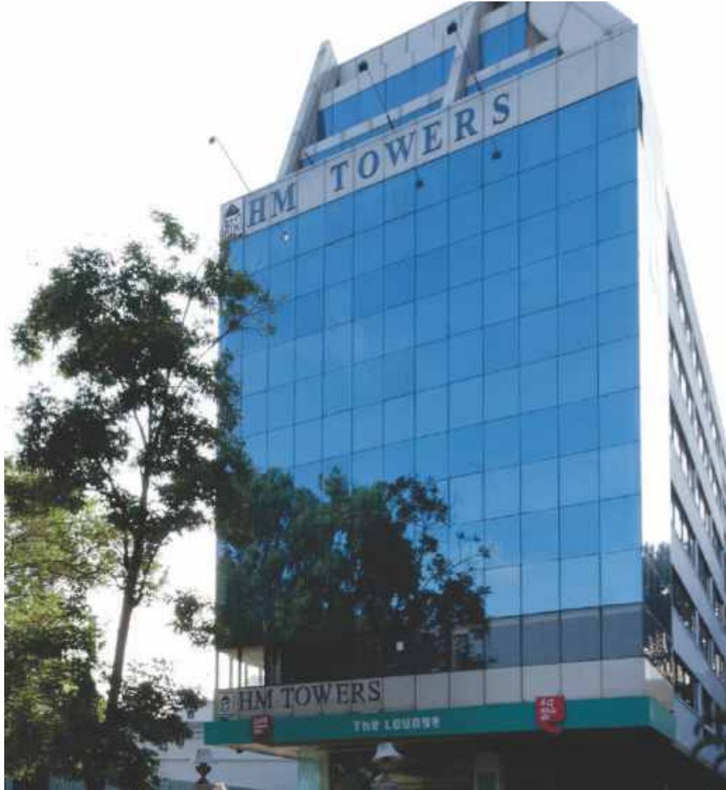
HM Towers Brigade Road
