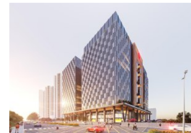
Western Windsor Park - Commercial
