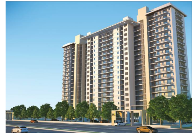
UNDER CONSTRUCTION GRAND CENTRA Sector 37 C, Gurgaon
