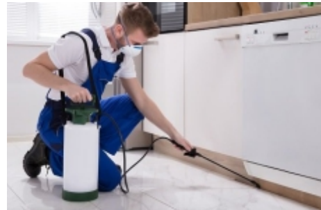
Anti termite treatment
