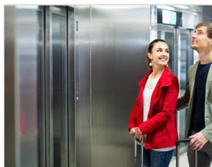
Passenger Lift With Power Back up
