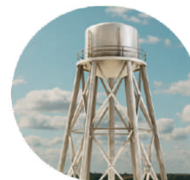
Over Head Water Tank
