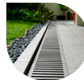
Rcc Steel Concrete Drainage
