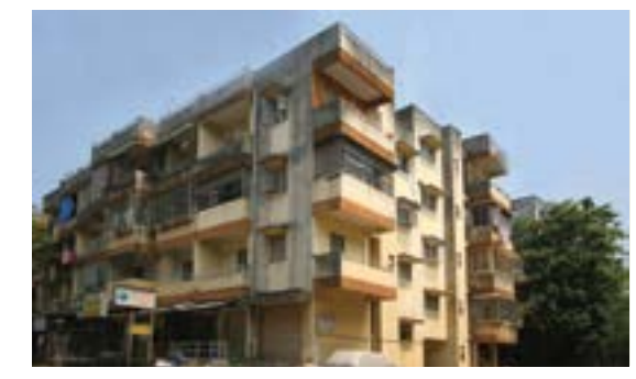
ANAND NAGAR 350 FLATS, PAUD ROAD
