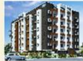
PANCHADURGA Residency Bappanadu, Mukky
