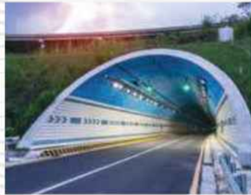
BORIVALI - THANE TUNNEL
